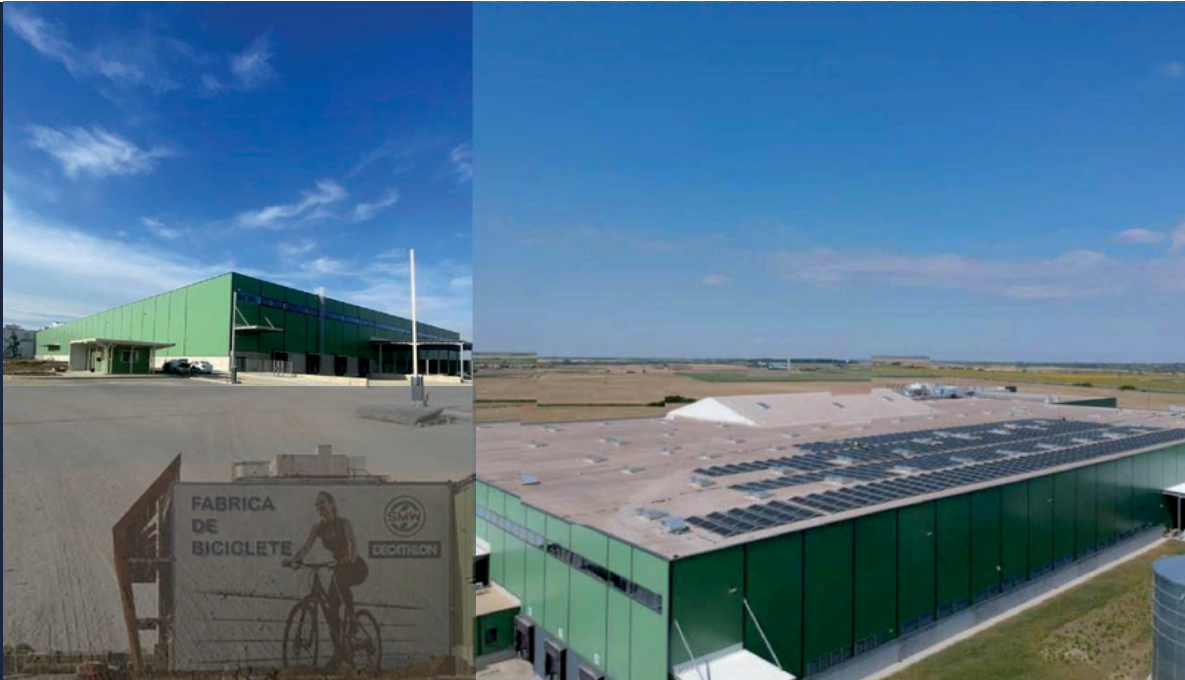
Sport Mechanical Work Shop srl Prosumator 525 kWp
